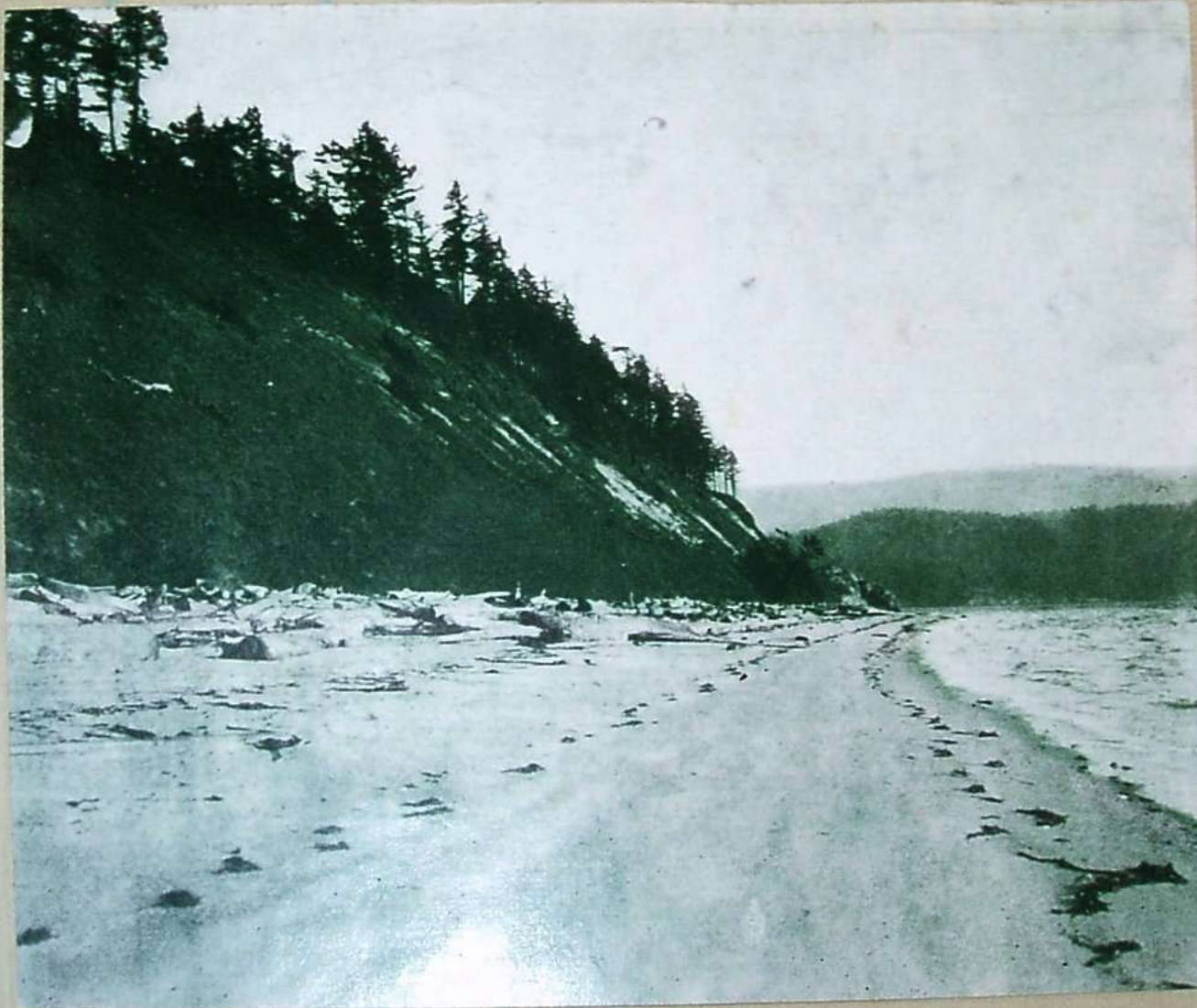
SOUTH SHORE, FACING VANCOUVER ISLAND
